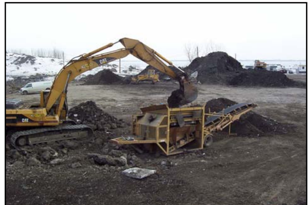
Plate 3: Removal of debris with a grizzly
