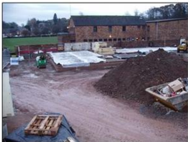
Plate 1 - Foundations of development being emplaced following installation of Envirotreat SMRBS
