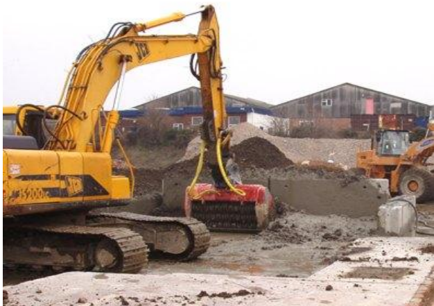
Figure 3 – Remediation of contaminated material.
