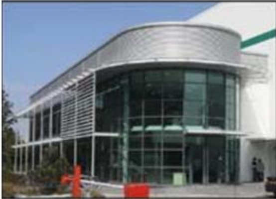
Plate 1 - Completed commercial buildings following the installation of the barrier.
