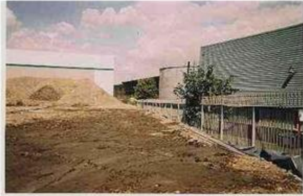
Plate 3 - The Re-active barrier following installation
