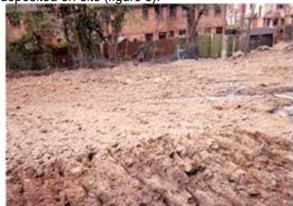
Figure 5 - Treated soils re-deposited on-site
