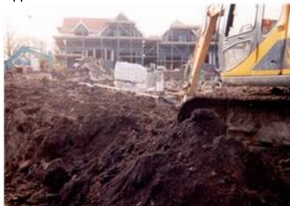
Figure 3: Excavation of contaminated soils in view of the new housing development.
