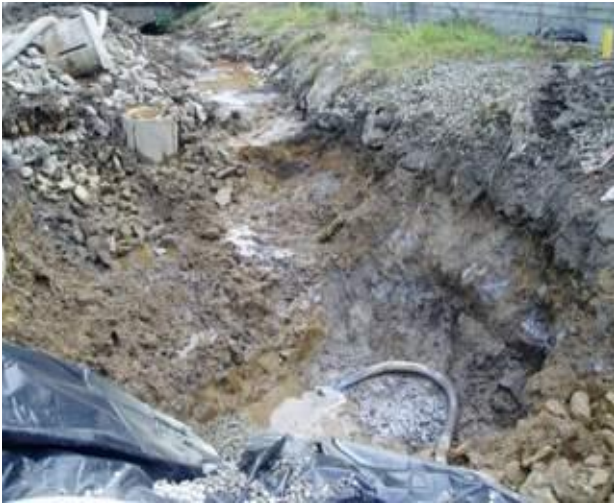
Plate 1 – Contaminated ground at Waterford.
