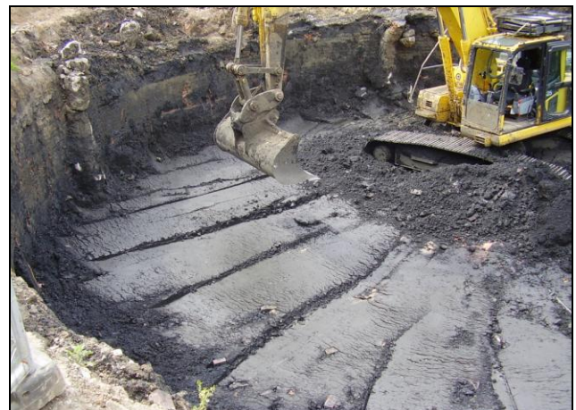
Plate 3 – Placement of treated soils into tar tank.
