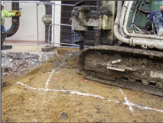
Plate 2 – Continuous Flight Auger installing soil mixed column.
