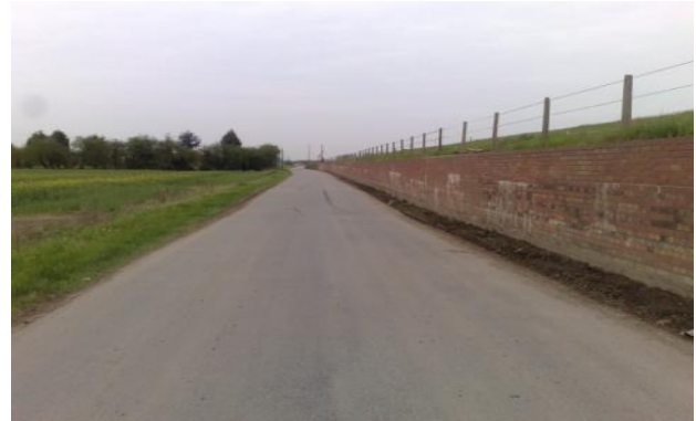
Figure 6 – Adjacent road following installation – significant improvement compared with Figure 2.
