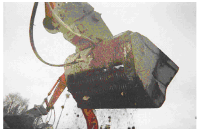
Plate 3: The processing bucket mixing contaminated soils with E-clay® slurry
