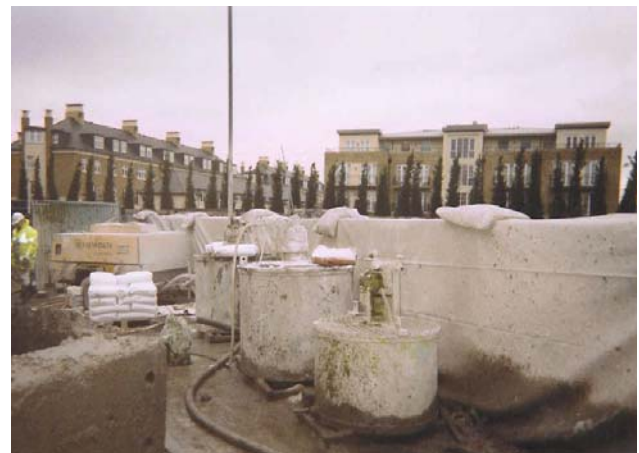
Plate 2: Set-up of the slurry production mixers
