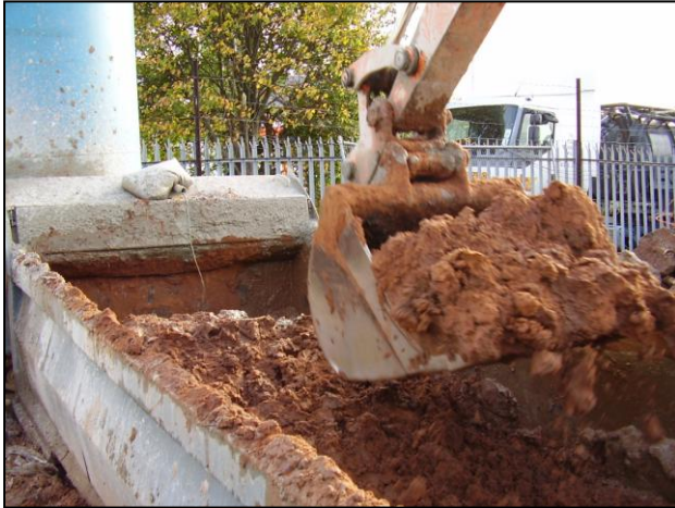
Plate 3- Contaminated soil being combined with E-Clay
