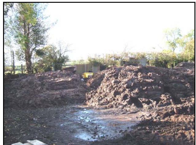
Plate 5 – Treated soils redeposited on-site awaiting site levelling.
