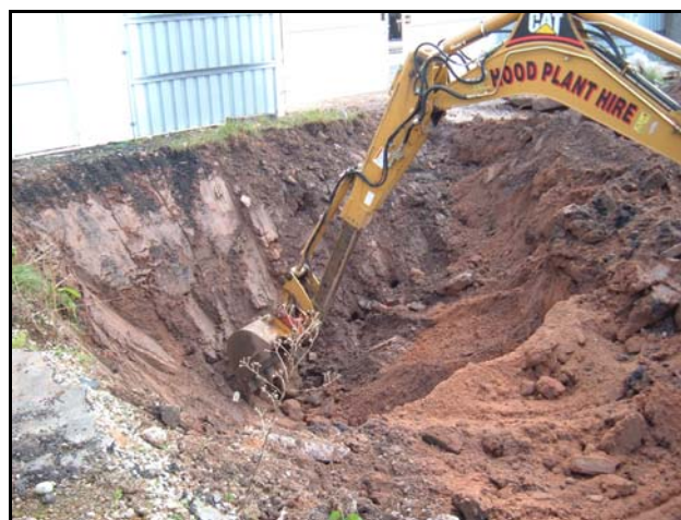
Plate 3 - Excavation of contaminated soils.
