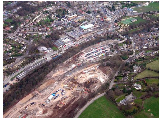
Plate 1 Area prior to development
