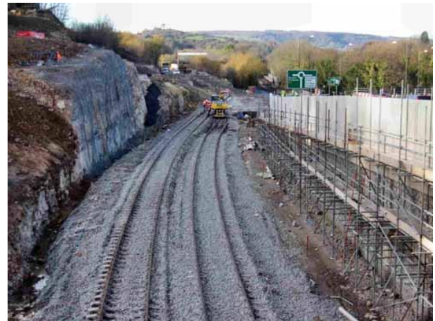
Plate 3 Treated material placed behind A6 bypass retaining wall
