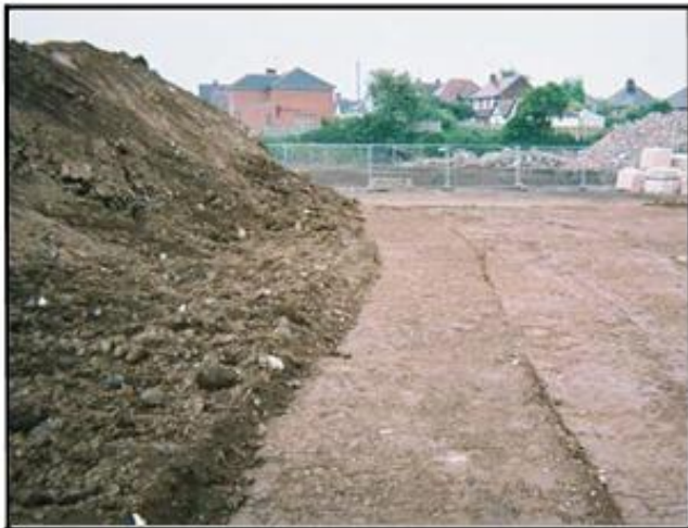
Plate 4 - Temporary stockpiling of the treated material
