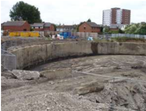
Figure 3 – Gasholder base following the removal of contaminated soils.
