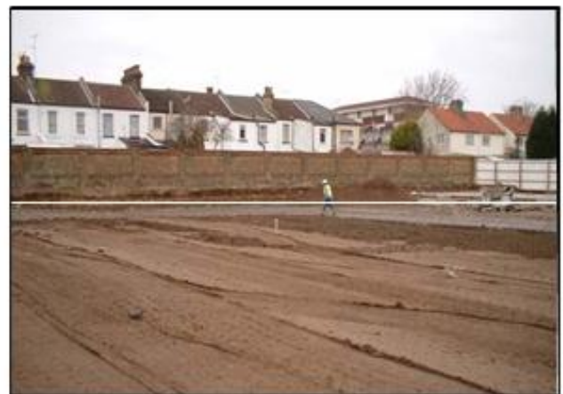
Photo 4 - Treated soils redeposited ready for the construction phase to begin.
