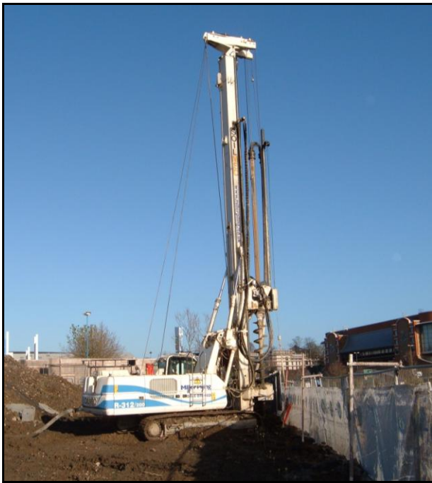
Plate 3: Barrier installation using a continuous flight auger
