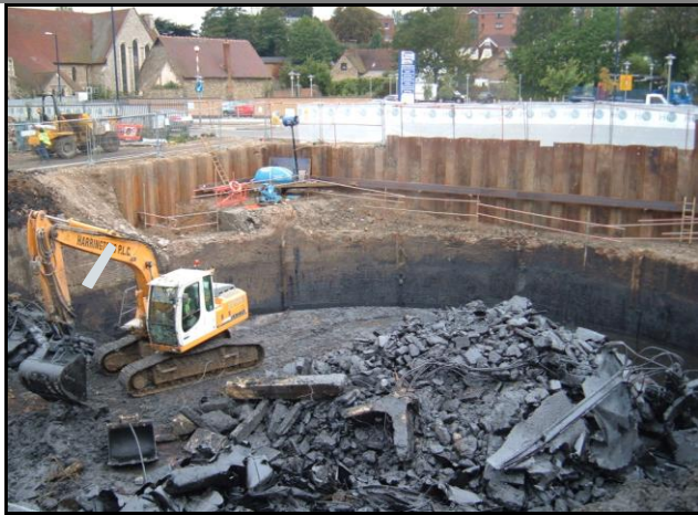
Plate 1: Excavation of the gasholder base
