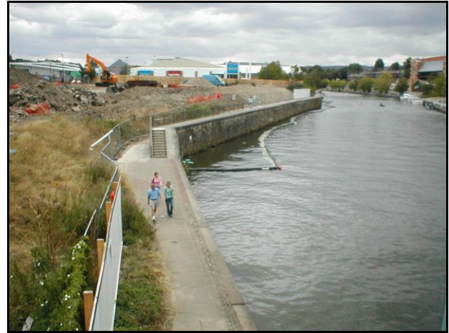
Plate 4: The main receptor the River Medway; floating spill booms were used as a precautionary measure.
