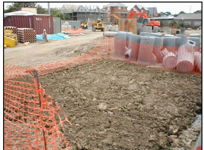
Plate 5: Contaminated hotspot backfilled with treated material.
