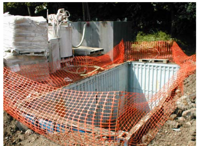
Plate 2: The mixing zone (foreground) and slurry production unit (background)
