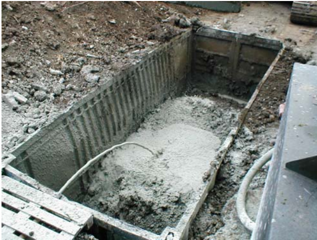
Plate 3: Combining the E-clay ® slurry with the contaminated soils
