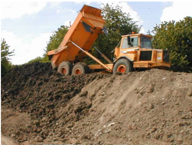
Plate 4 – Temporary stockpiling of the treated material
