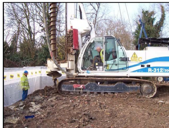
Plate 3 SMRBS installation
