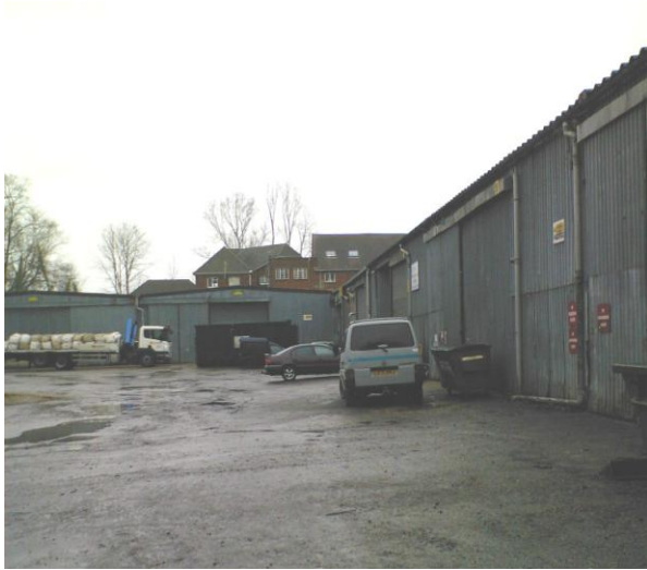
Figure 1 - Site Prior to Remediation
