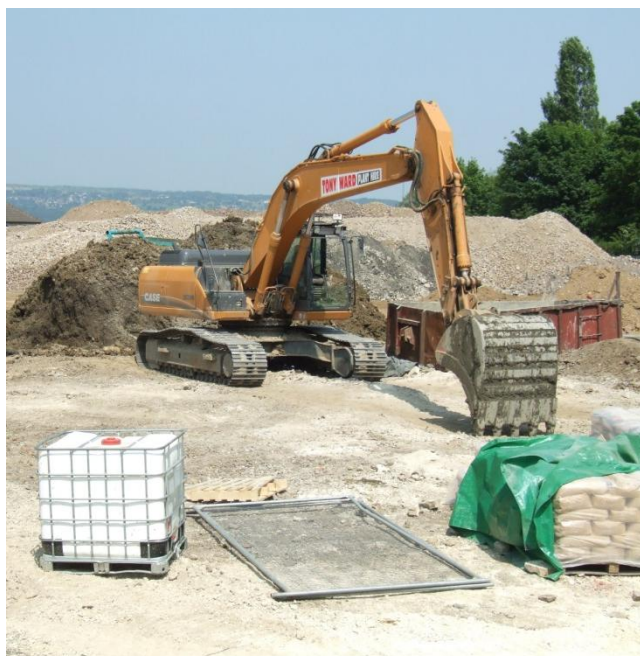
Figure 3 - Onsite treatment operation.
