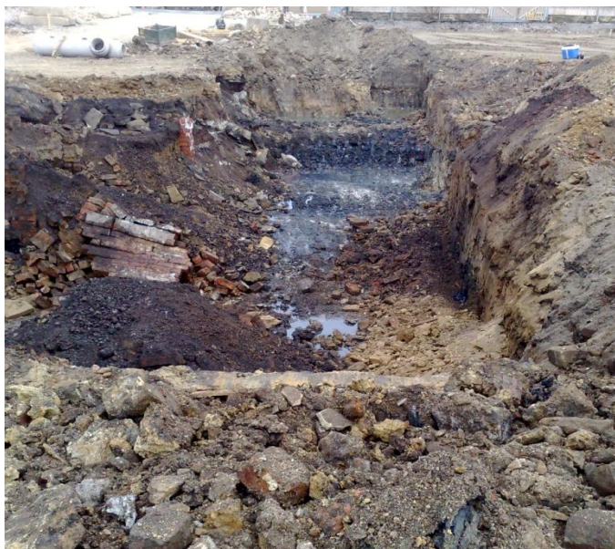
Figure 1 - Site prior to remediation
