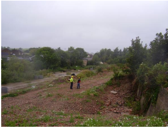
Figure 1 - Site prior to remediation
