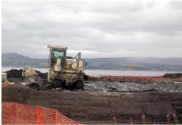
Figure 3 WIRTGEN blending E-Clay and contaminated material.
