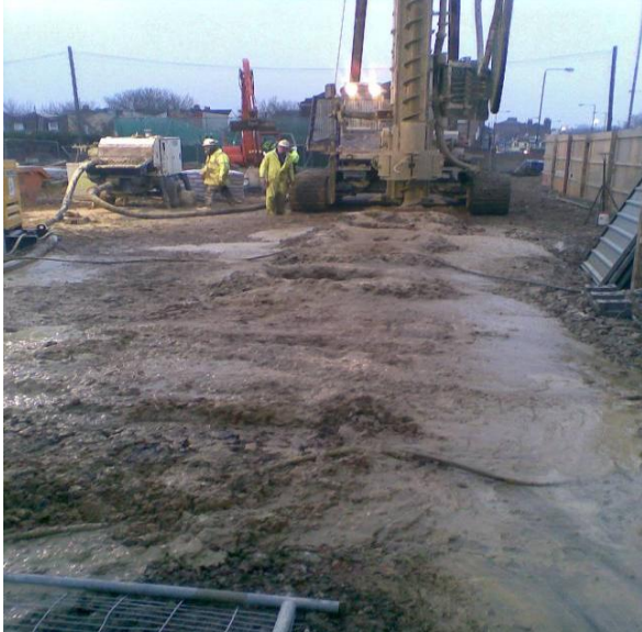
Plate 2 – Installing barrier using Auger piling rig.
