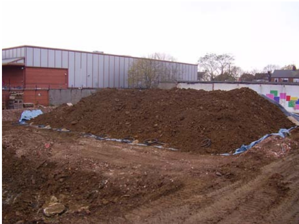
Plate 3 Complete biopile prior to covering
