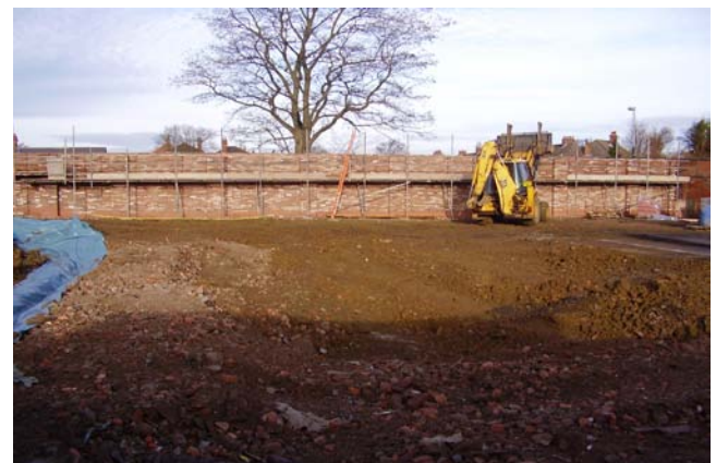
Plate 4 Redeposition of the treated material.
