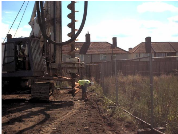
Figure 2. Installing the barrier using continuous auger piling.
