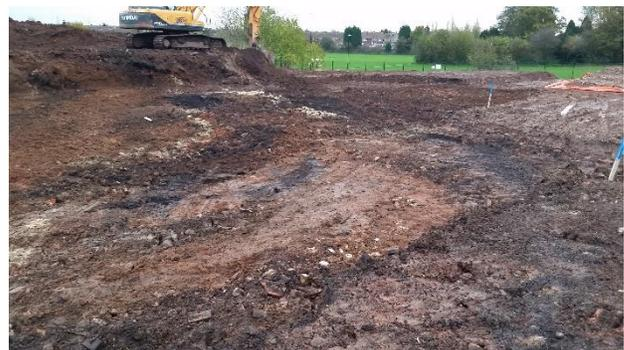
A crucial element of these works was the assessment of excavated soils generated as part of the cut & fill and enabling works for suitability for reuse on site or placement in the proposed burrow pit in the North East of the site.
