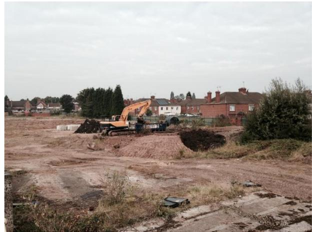
These works were undertaken in September of 2014. In total as estimated 1,250m<sup>3</sup> of soils were treated.
