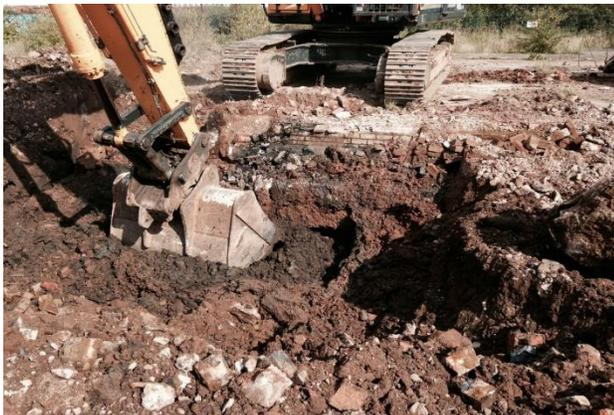
Stockpiled soils were treated using a suitable E-Clay formulation specific to the the respective contamination within the soils.
