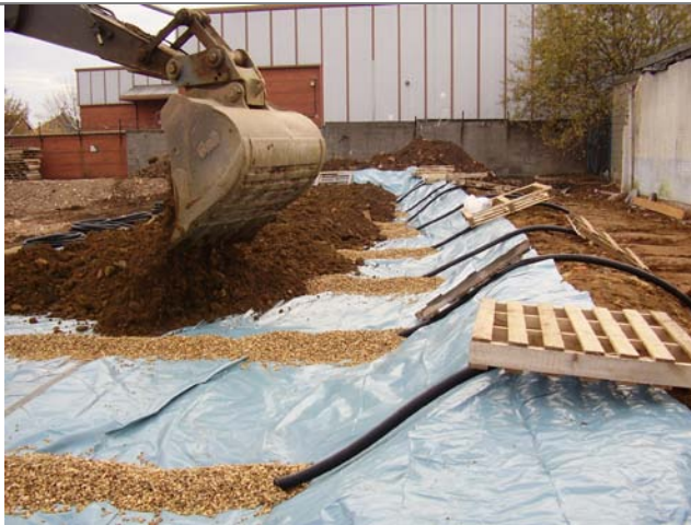
Plate 2 Biopile construction
