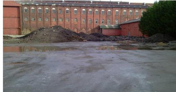
The treatment strategy was therefore to enable a waste recovery process to be implemented, producing a treated material which could be utilised on site as a substitute for imported fill.
