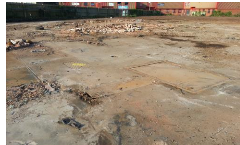
Figure 3 – Southern Area of the Site Following Demolition
