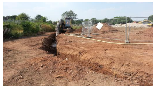
Figure 5 – In-situ Installation of E-Clay Permeable Reactive Barrier
