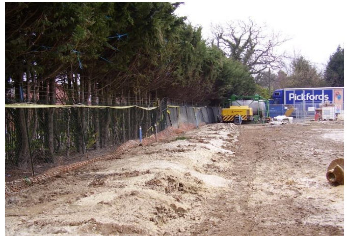
Figure 3 – Line of the installed barrier.
