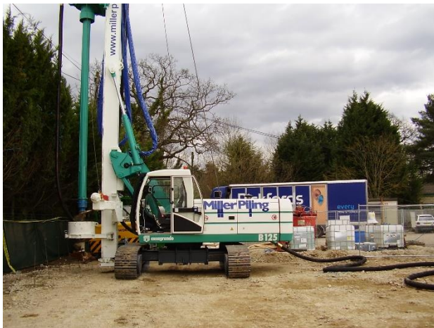
Figure 2 – The piling rig and auger.
