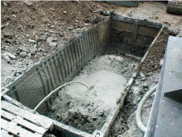
Plate 3: Combining the E-clay<sup>®</sup> slurry with the contaminated soils
