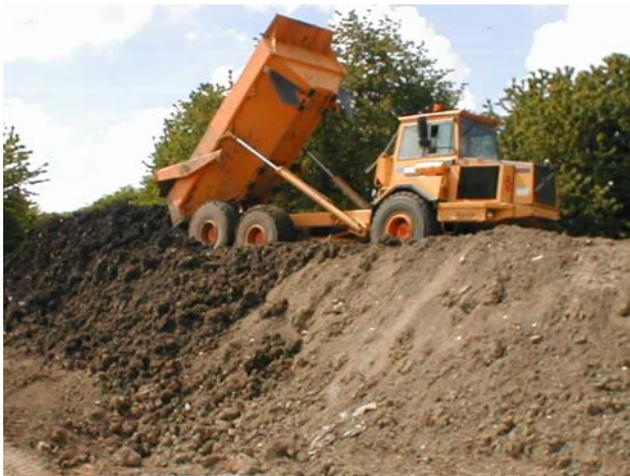
Plate 4 – Temporary stockpiling of the treated material
