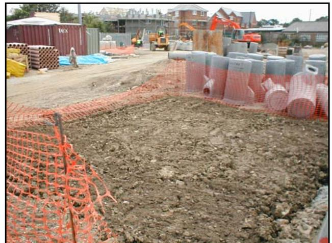
Plate 5: Contaminated hotspot backfilled with treated material.
