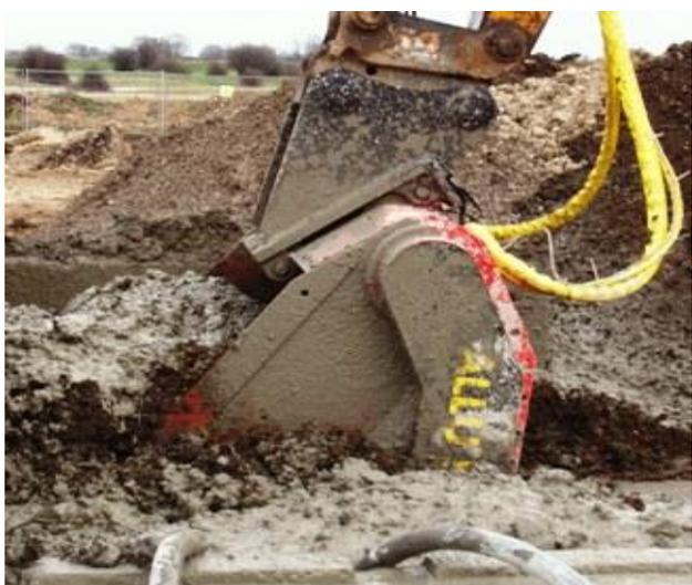
Figure 4 – Mixing of clayey soils with E-Clay (grey coloured slurry) using the specialist processing bucket attachment on a conventional excavator.
