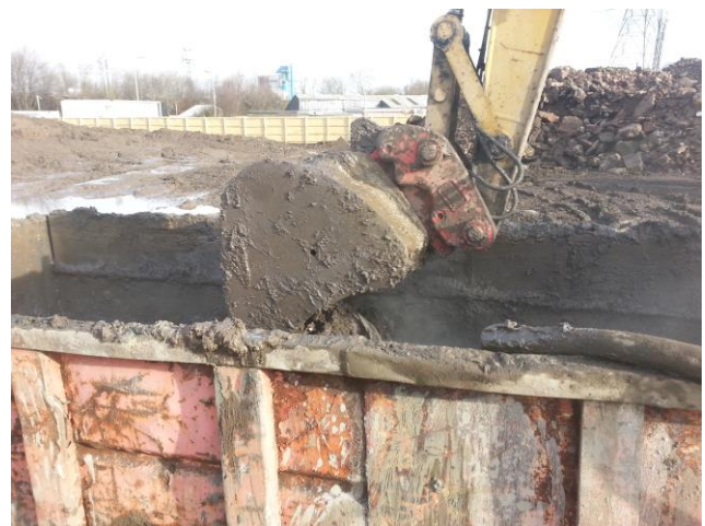
Figure 6 – Ex-Situ Treatment of Contaminated Soils
