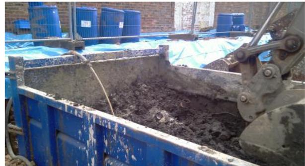
The treated soils were stockpiled and allowed to fully cure. Validation samples were submitted to accredited laboratories for leachate analysis to confirm compliance with the designated RTC. All TPH leachate results were <10ug/l demonstrating full compliance with the 500ug/l target value.
