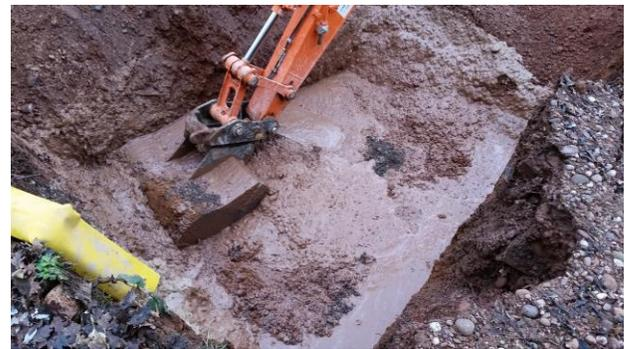
Previously set aside un-contaminated soils (reduced dig) were reinstated.
