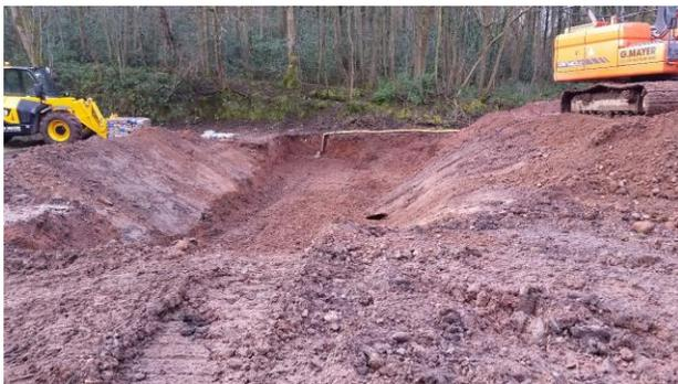
The delineated area was reduced in depth to above the contamination, the area was subdivided into sections to enable assessment of required volumes. Within each section pre-determined volumes of E-Clay slurry were added and soil mixed to the required depth. Each section was treated in turn until the whole delineated area had been treated with E-Clay treatment slurry.
