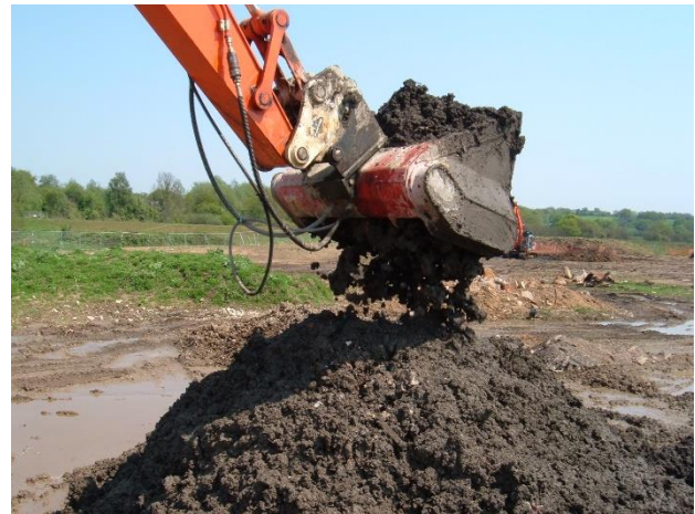
Figure 6 – The stabilised / solidified soils
