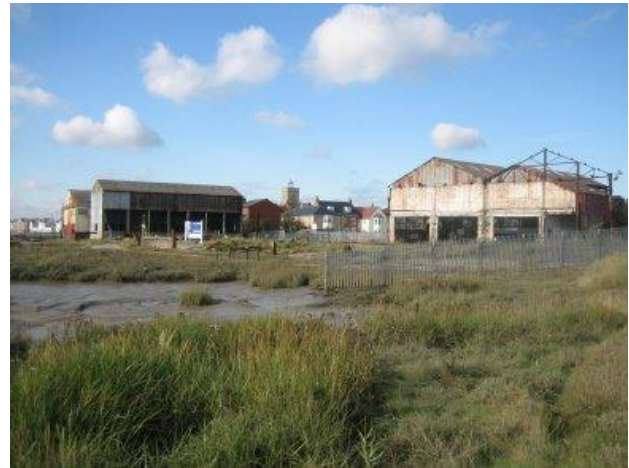
Figure 1 – The site prior to Remediation
