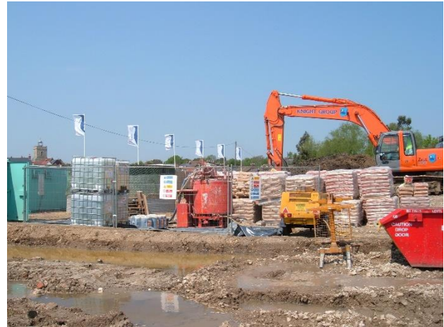
Figure 2 – Treatment Area Set Up
