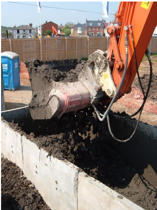
Figure 5 – The ex-situ mixing operation
