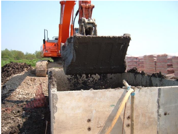
Figure 4 – The ex-situ mixing operation
