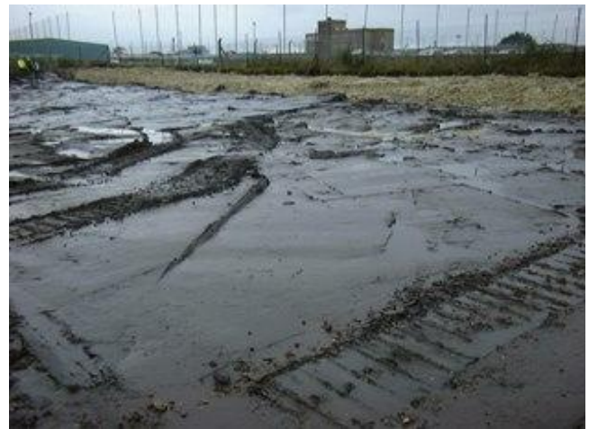
Plate 3 – Compacted treated material re-used as infill.
