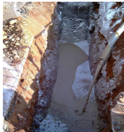
Figure 7 – Addition of E-Clay / Reductive Additive
