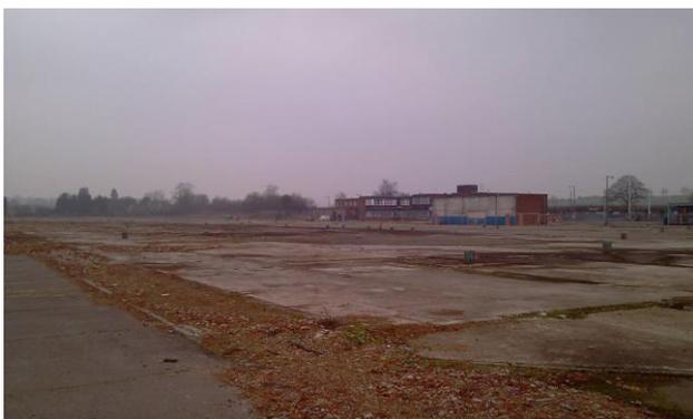
The prime environmental receptor was identified as the Rothley Brook, located approximately 100m south of the site. Human health protection is provided by means of the warehouse concrete base (the hardstanding being an effective pathway break).
