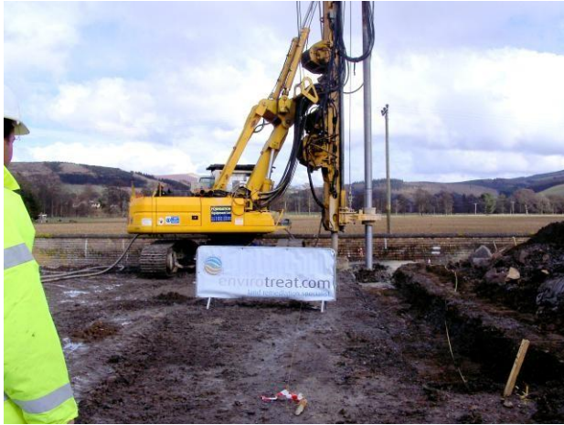
Plate 4 - Barrier Installation utilising a Carillion Piling CFA Rig and Expertise
