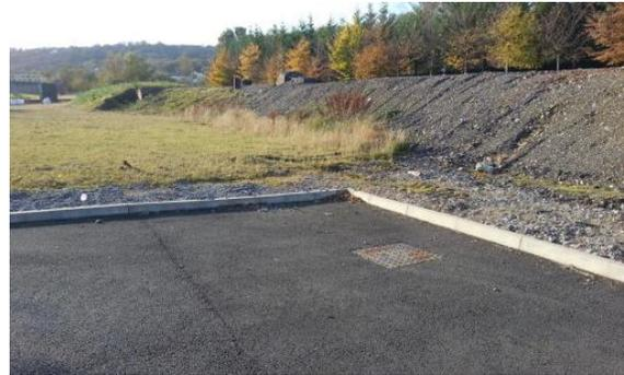
The inert oversize concrete materials were crushed and reused to raise levels in an area prone to flooding (due to a slight depression). This area is shown in Figure 5 below.
