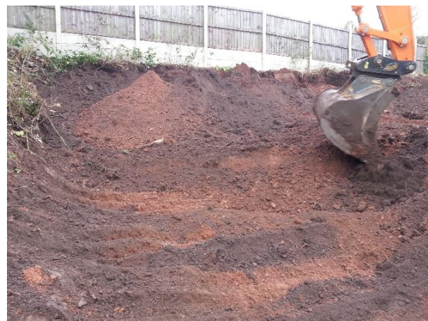
Figure 2 – Excavation of bulk JKW contamination.
