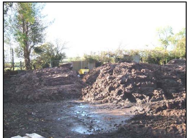
Plate 5 – Treated soils redeposited on-site awaiting site levelling.
