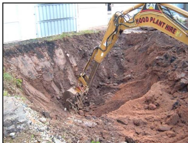
Plate 3 - Excavation of contaminated soils.
