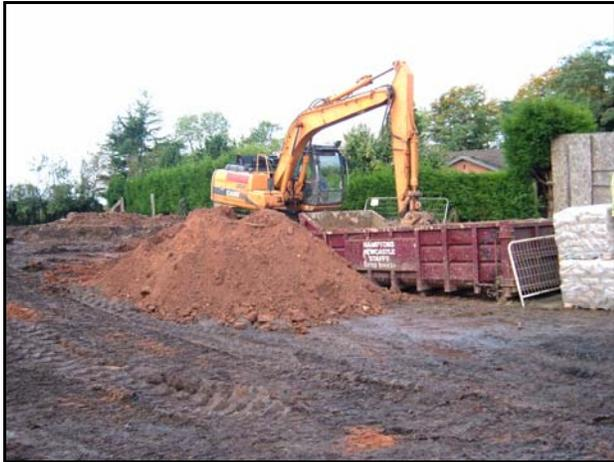
Plate 4 - Set-up of the excavator and skip to mix the contaminated soils with the E-clay<sup>®</sup> slurry.
