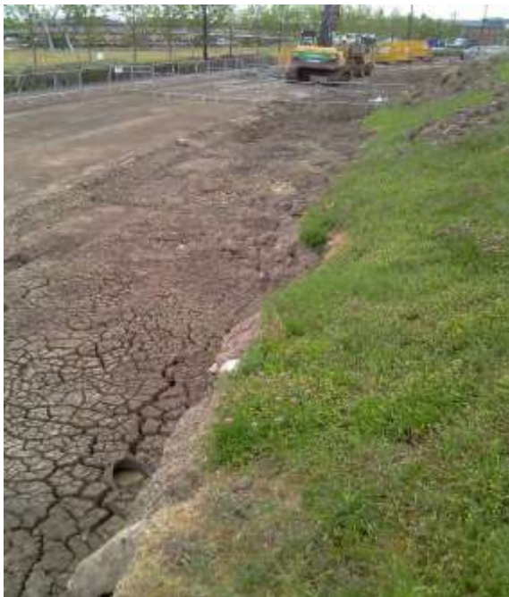
Figure 2 – Installed Reactive Barrier
