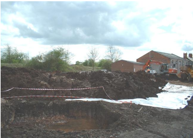
Plate 3 – Temporary stockpiling of the treated material
