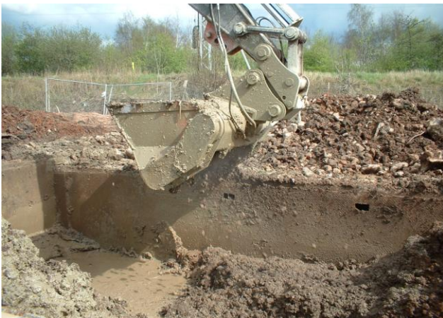
Plate 2: The processing bucket mixing contaminated soils with E-clay® slurry
