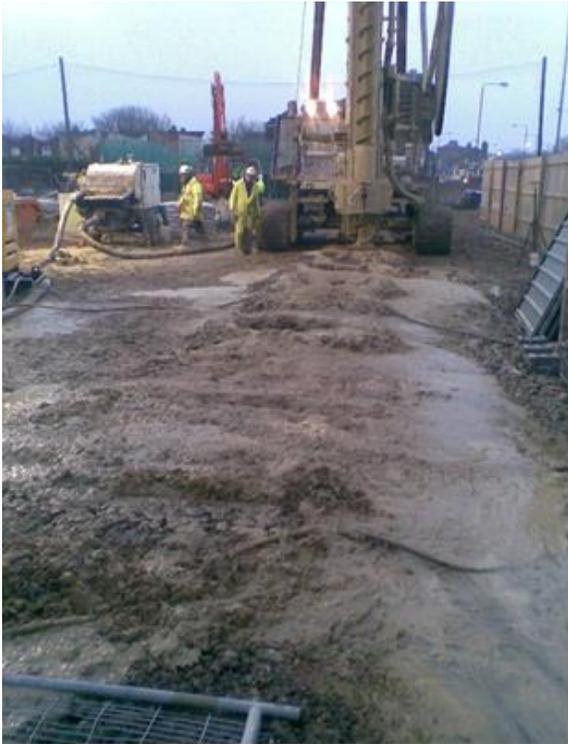
The reactive barrier section comprised of a triple row of overlapping columns as shown in Figure 4 below.
