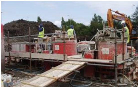
The E-Clay slurry was pumped across to the mixing zone. The contaminated soils were then treated in the mixing zone by adding the designated volumes / amounts of E-Clay slurry and cementitious materials to the contaminated soils (see Figure 4 below). The treatment materials and soils were then mixed in 10m<sup>3</sup> batches to produce a homogeneous treated [E-Clay Stabilised] material utilising excavators mounted with conventional buckets as shown in Figure 5 below.
