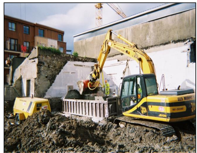
Plate 2 – Remediation of site using 'allu' bucket.
