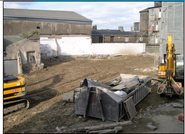
Plate 4 – Treated soils re-deposited ready for the construction phase to begin.
