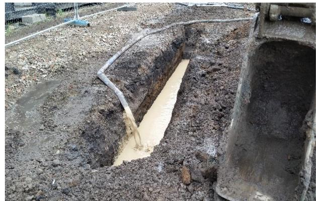
Figure 3 – Delivery of E-Clay Slurry to the Barrier Installation
