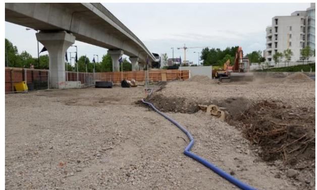
The barrier was installed to a maximum depth of 3.2m bgl in accordance with the prevailing site geology observed along the barrier alignment.
