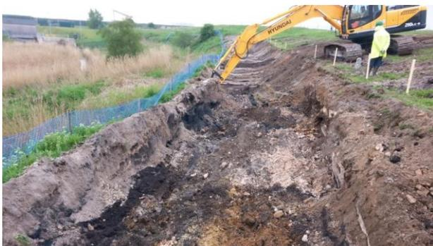
Figure 6 – *Ex-Situ* Treatment of Gas Works / Spent Oxide Waste in Area 9
