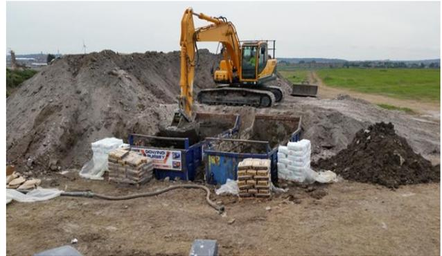
The spent oxide waste on the adjoining site (Area 7) was delineated by the excavation of a number of trial pits. The identified area was treated *in-situ* treatment utilising the designated stabilisation medium incorporating cementitious materials, the appropriate E-Clay formulation and specialist additives. The contaminated material in Area 7 was predominantly spent oxide waste with an associated very low pH necessitating a different stabilisation medium to that employed in Area 9.
